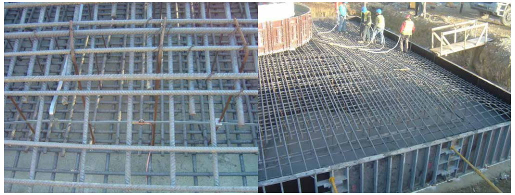
Image 13: Earthing system of a wind power plant
